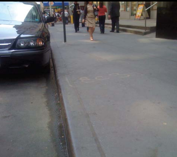
Standard Concrete Curb (with steel face)
